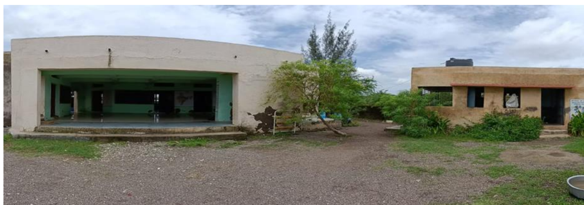
Figure 4: Infrastructure of the school in Bhachadar village
