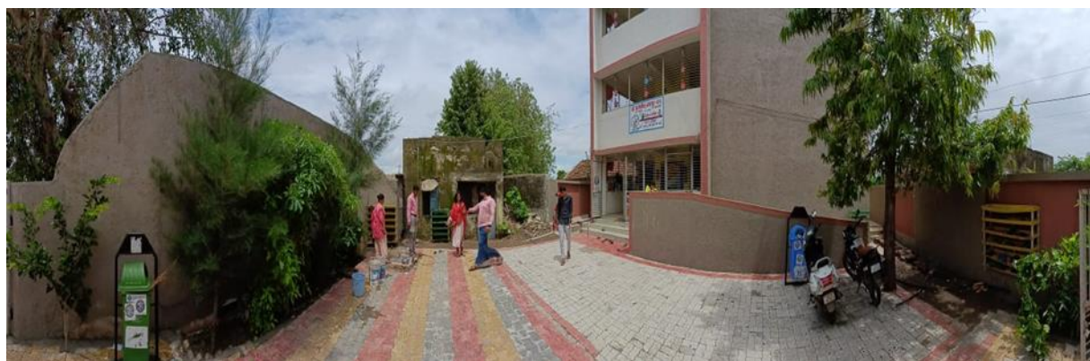
Figure 13: Infrastructure of the school in Vad village
